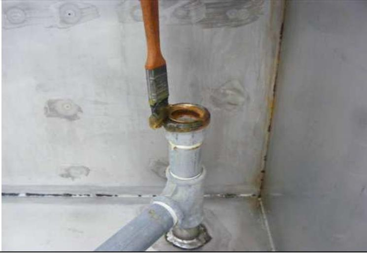
**Limpe** bem as conexões as roscas e lubrifique antes de montar.
